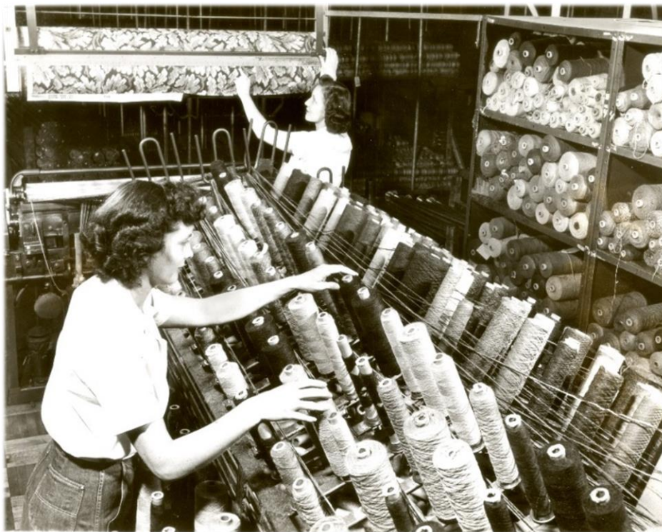
Figure 20: During the latter part of the bedspread industry's boom complex machines had been incorporated in order to increase productivity. These machines paved the way for the carpet industry which utilized similarly engineered, but much larger, equipment. *Photo Courtesy of the Bandy Heritage Center
