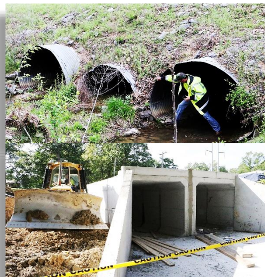
Figure 20: Before and after of a culvert replacement on Beaverdale Rd. where Whitfield County saved approximately $300,00 by utilizing its on public works department rather than a contractor
